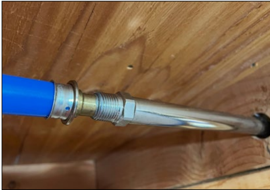
Figure 9.46 PEX Connected to a Hose Bibb/Wall Hydrant
