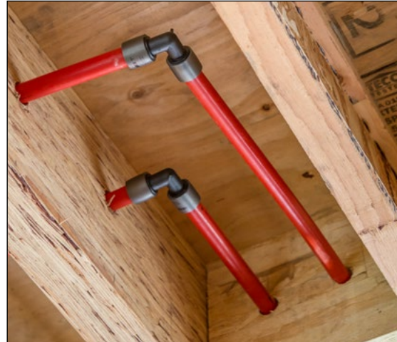
Figure 9.6 Elbow Fittings in a Confined Joist Cavity
