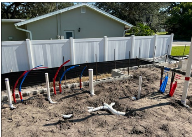
Figure 9.28 PEX Installed in Ground Below a Future Slab
