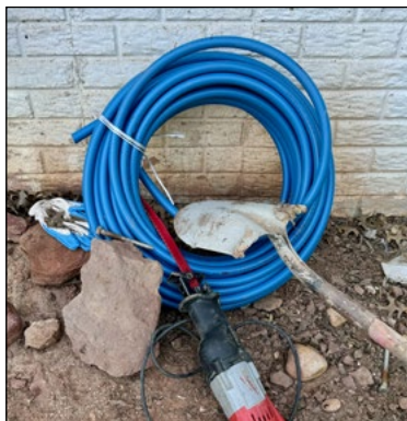
Figure 9.2 Sharp Objects Can Damage PEX
