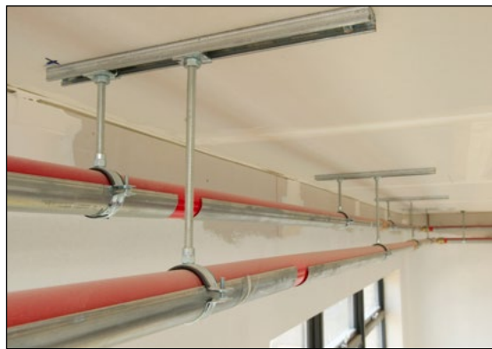
Figure 9.10 Pipe Support Channel
